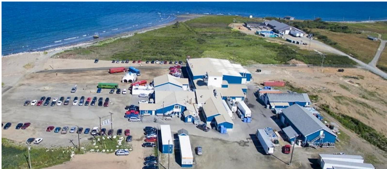
Figure 14: Champlain Seafood Processing Plant (now closed)
